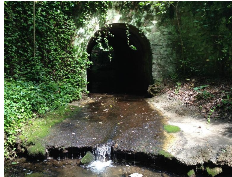
Drainage features under roadway crossings provide historic interest.
