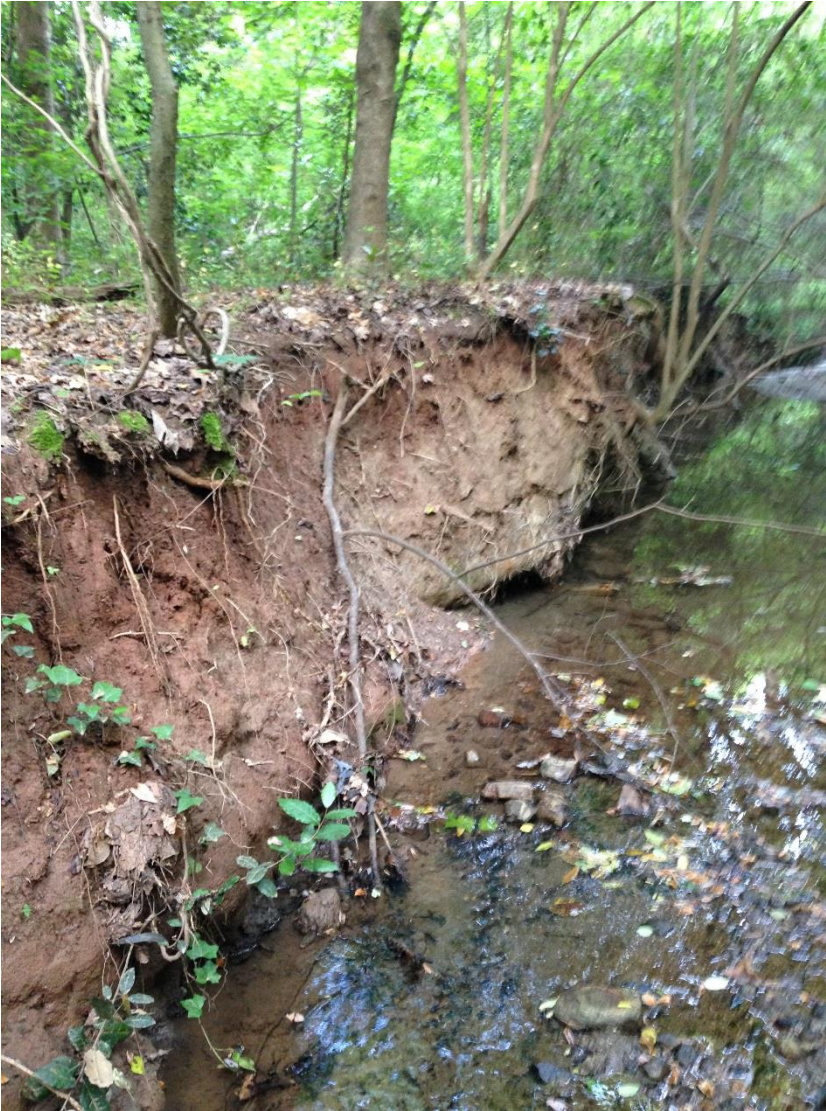
Existing erosion observed on site.
